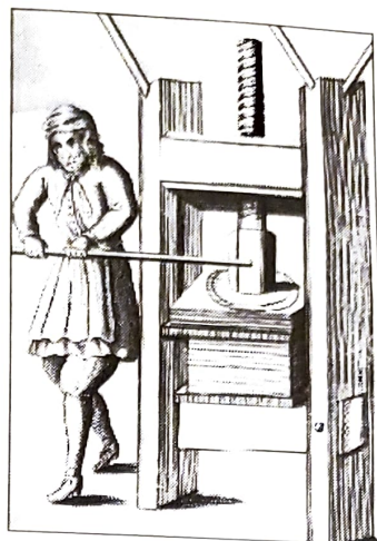
The large jackscrew on a printing press
